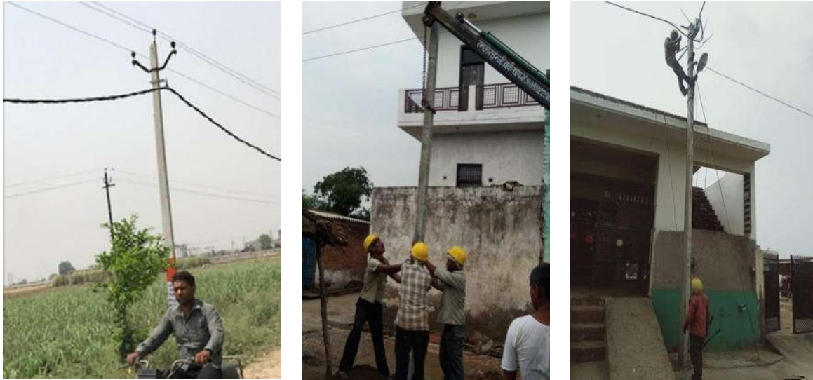
Photo 1: ABC Installation and Stringing Work
